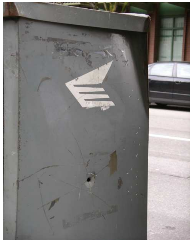
East side relay box with bullet hole, presumably used as target practice!
